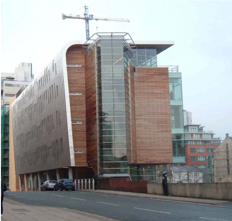
A building with an unconventional form creates interest in the urban fabric, Piccadilly Basin, Manchester.
