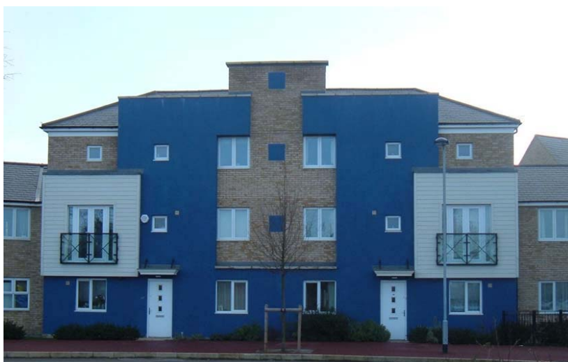
The use of colour emphasises the shapes created in the design of the building elevation. Orchard Park.
