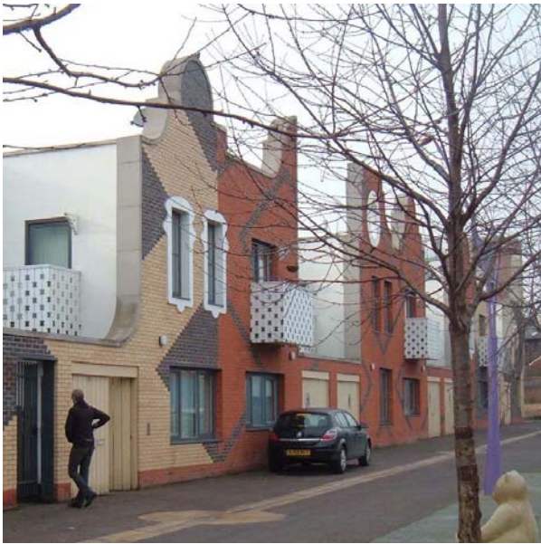
Buildings designed to break the symmetry of the front elevation to ensure future personalisation or alterations by residents will not visually unbalance the elevation. New Islington, Manchester.
