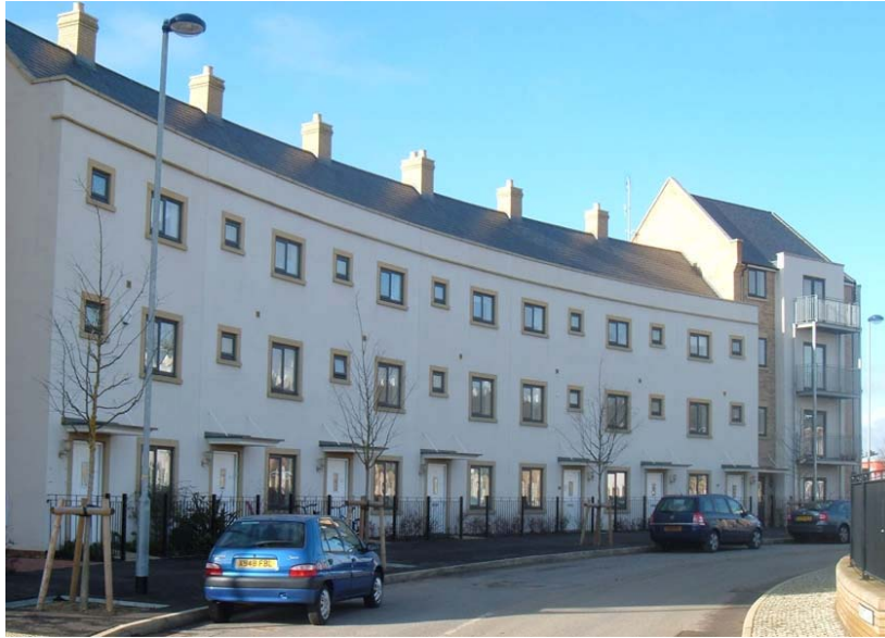
The size, shape and alignment of windows on a plain background of the building elevation, creates a primarily horizontal emphasis, giving the impression of a long low terrace. Orchard Park.
