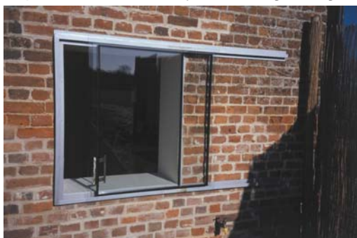
Contemporary sliding metal window applied to surface of existing brickwork wall, separating new materials and elements from old, clearly showing the building's evolution (Hudson Architects)
