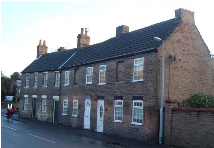
Blind windows used to continue the rhythm of openings in the façade of a terrace. St. Neots.
