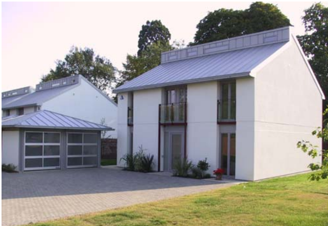
Infill houses, Melbourn. The rendered walls and tall window proportions make reference to the listed house, with contemporary metal roofing and window frames (Plum Developments).
