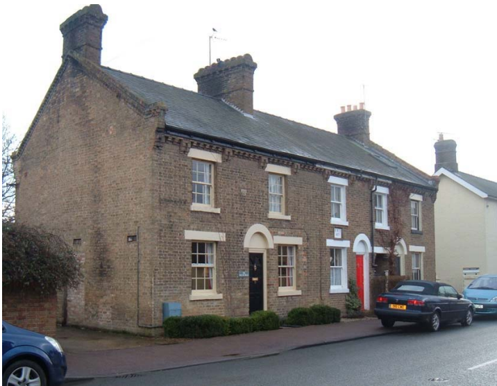
A rhythm of openings in an elevation unifies a terrace of varied built forms. Cottenham.
