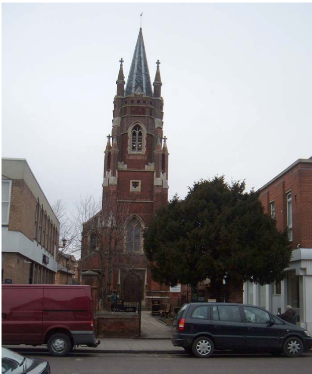
7. On the left hand side an opening in the built form fronting the street provides a view of the second church front with its spire.
